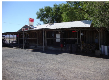
Middlegate Station Nevada
